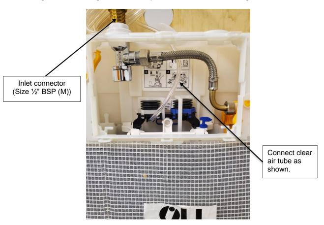
Figure 4: Inlet hose and air tube configuration
