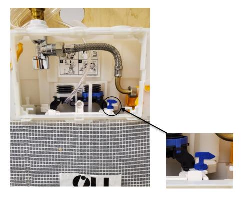
Figure 5: Inlet hose and air tube configuration
